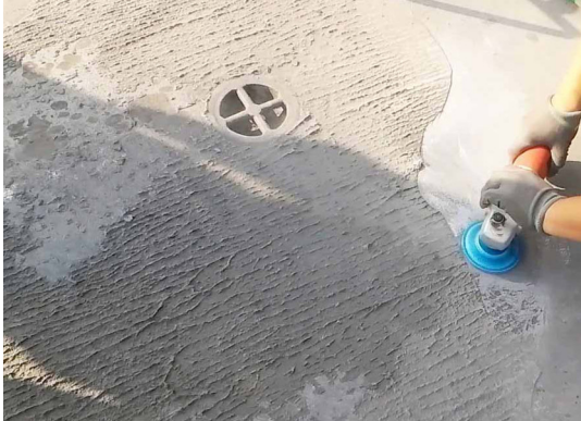
Tool in use on a concrete surface
