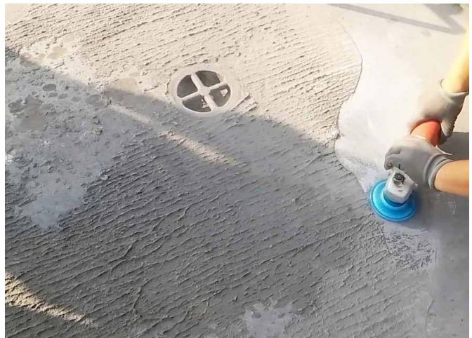
Coating removal with NON-SKID CUP: qualitative application photograph.
