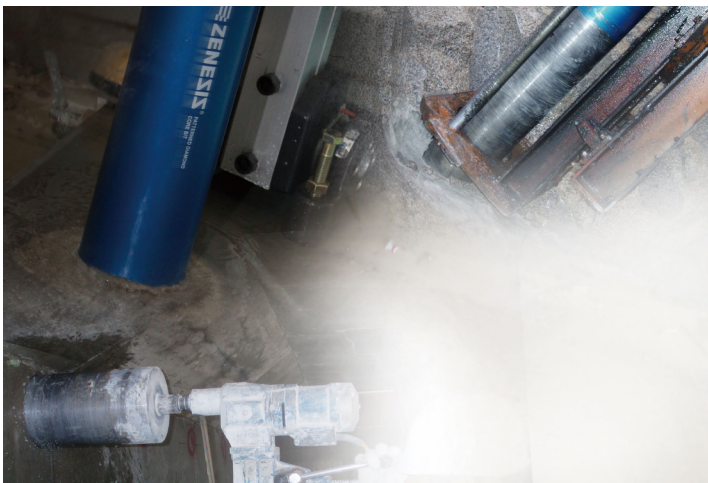
Construction: drilling - Application
