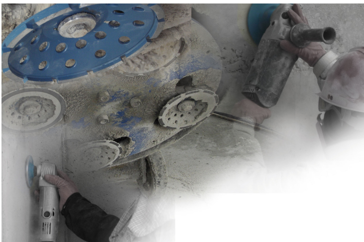
Construction: grinding and polishing - Application
