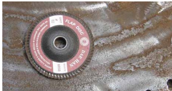
Rust removal: flap disc.
