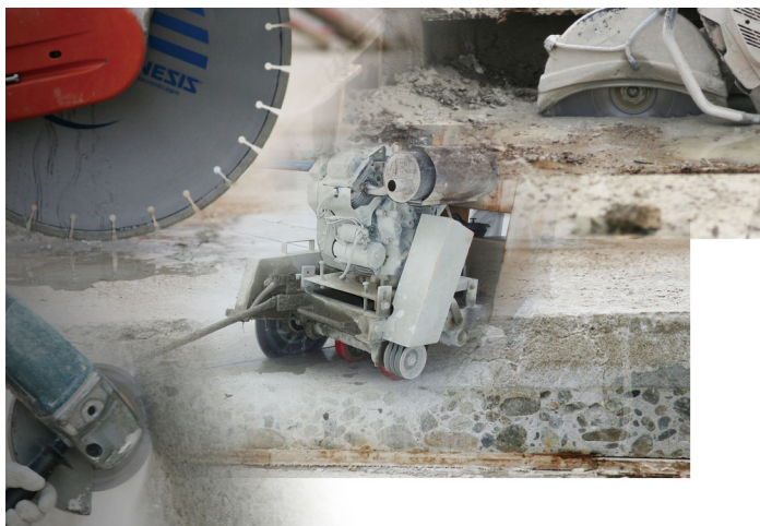
Construction: sawing - Application
